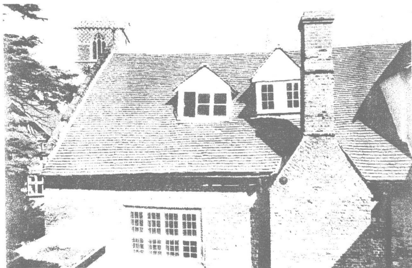
Roofscape after restoration.
