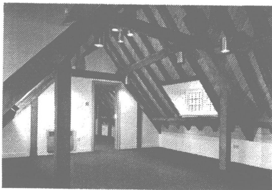
View of upper floor after restoration.
