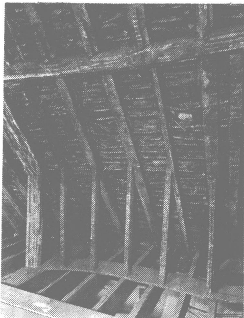
View of the roof during restoration.
